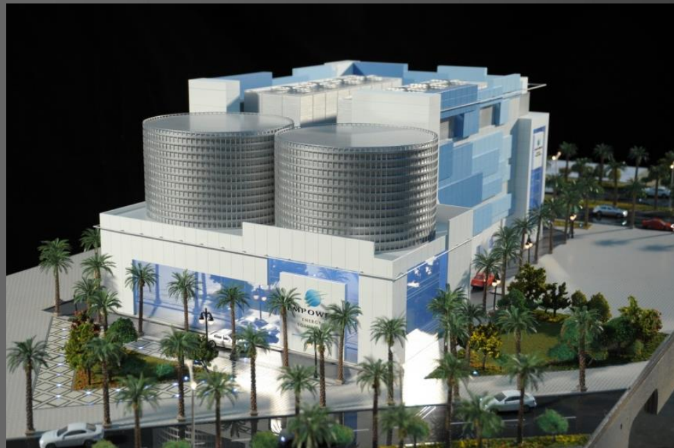
Thermal Storage units in Empower's Business Bay District Cooling Plant
